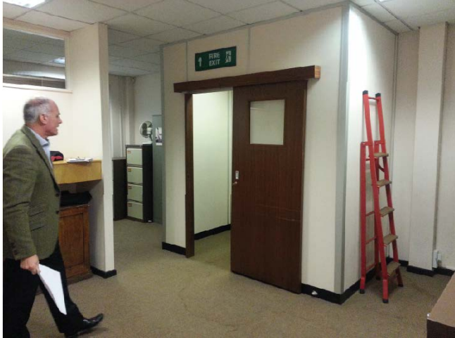
Conference room - before
