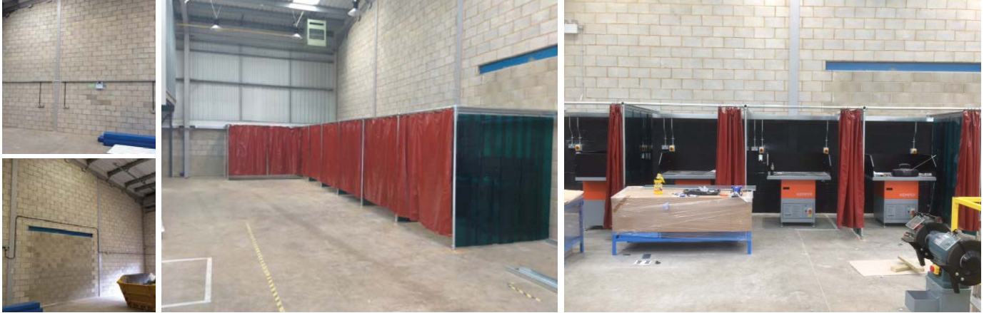
Installation of new welding bays.
