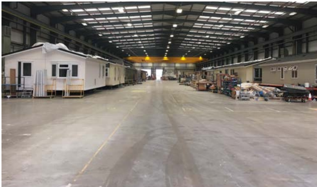
Before: The production facility at Prestige and Homeseeker Park and Leisure Homes in Rushden before the industrial mezzanine was installed.
