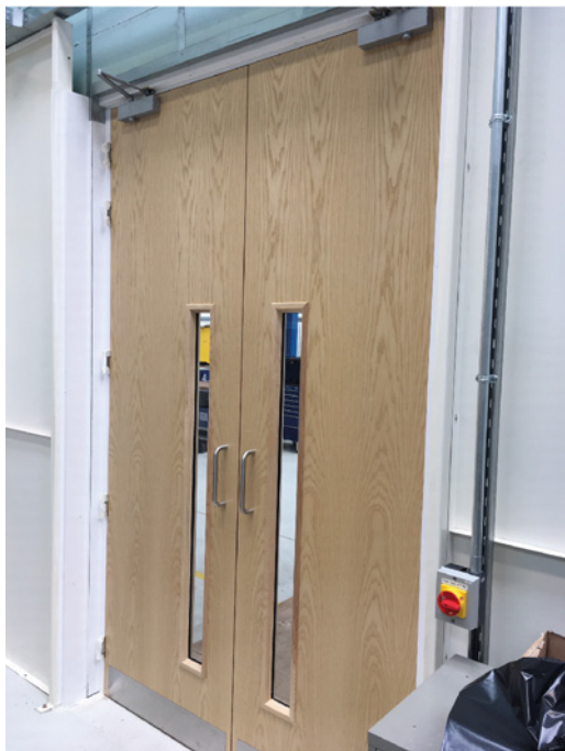
Close up of the double door set with acoustic seals and vision panels.
