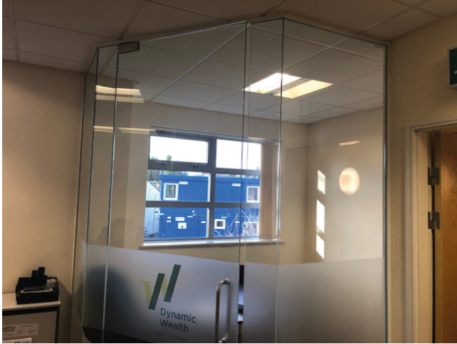
Upstairs - corner office with single glazed glass partitioning (before)
