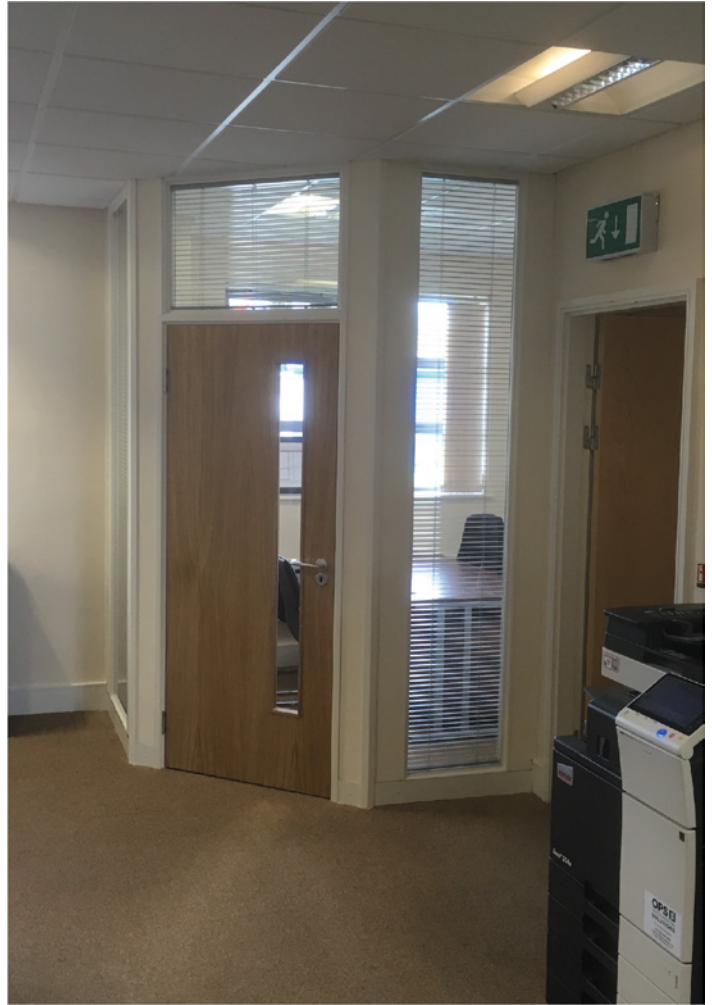
Upstairs - double glazed partitioning with privacy blinds now installed (after)
