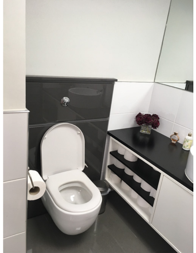
After: the customer manufactured the high spec toilet cubicles in-house
