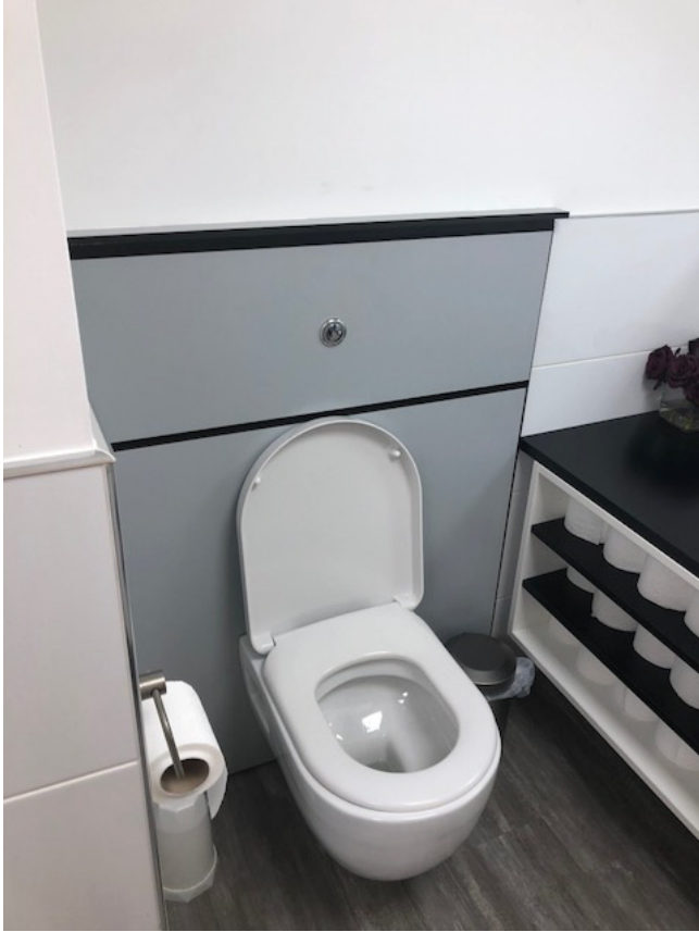
Ladies Toilets - Before
