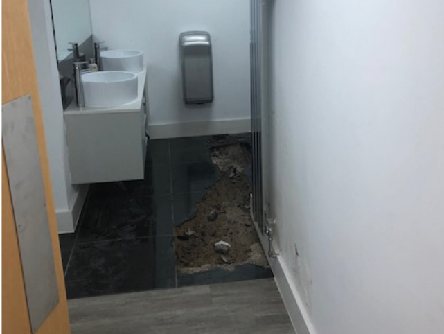
Gents Toilets - Before
